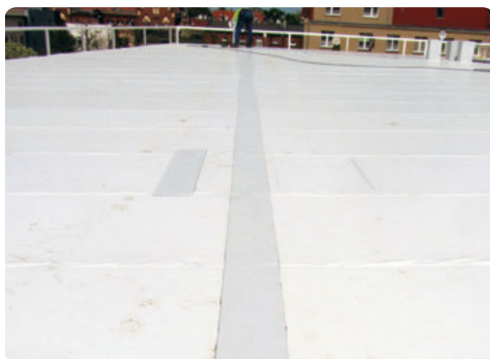
Transverse panel joint covered by welded FLAGON SV membrane strip
