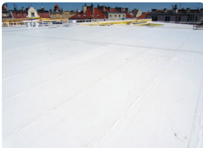
View of the roof
