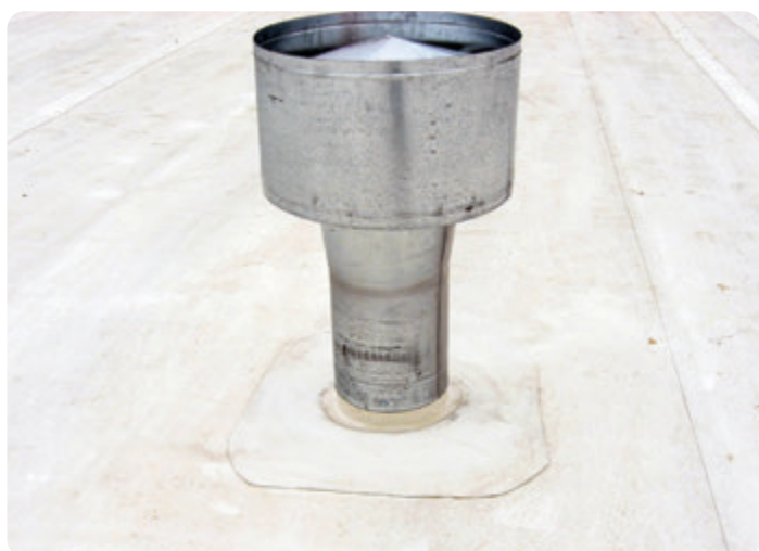
Tooling of ventilation channel
